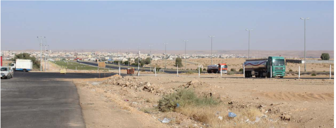
Figure 10-5: Typical Settlement within the Settled Desert Plain LCT
