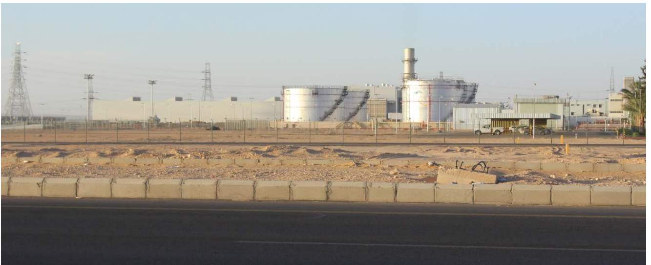
Figure 10-6: Industrial Land Use within the Settled Desert Plain LCT (Al Jouf Power Station)
